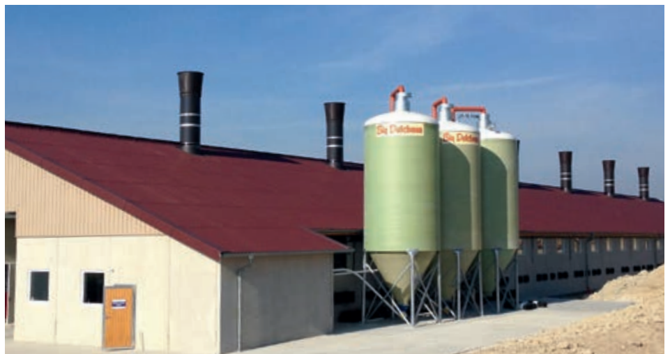
Example: exhaust air exits > 3 m above ridge
